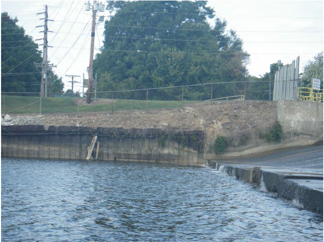
Figure 8. Area of localized very high erosion risk in the bypass reach area
